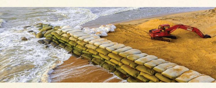
WAVEPLUS Geobags are specially designed to resist sea erosion and to preserve the beaches. These bags are extremely durable in the marine environment, exposed to heavy sunlight.
